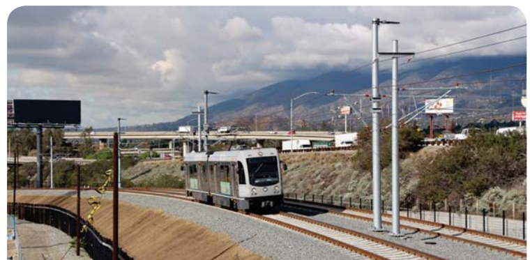
During a functional test of the Traction Power Systems in Duarte as it approached the San Gabriel River in Irwindale, a two-car Light Rail Vehicle (LRV) is seen here traveling quietly and effortlessly under its own power.
