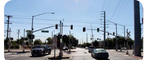
Recently completed Mountain Ave grade crossing, bordering the cities of Duarte and Monrovia, now with dedicated right and left turn lanes, but missing the large hump and sharp turn in the road.
