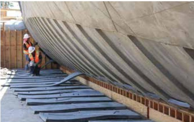
The bridge's ribbed design was created by fastening polymeric form liners onto curved forms. Here, workers pull the liners from the concrete
